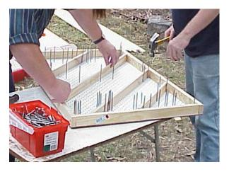
Place the second peg board over the nails and press it down. Make sure the holes of both peg boards are lined up (the nails will ensure this). Screw both peg boards to the edge and middle battens (one screw per side and one screw per middle batten will do, for each peg board). These are just to hold things in place - more screws will be added through the plywood sheet at the end.
